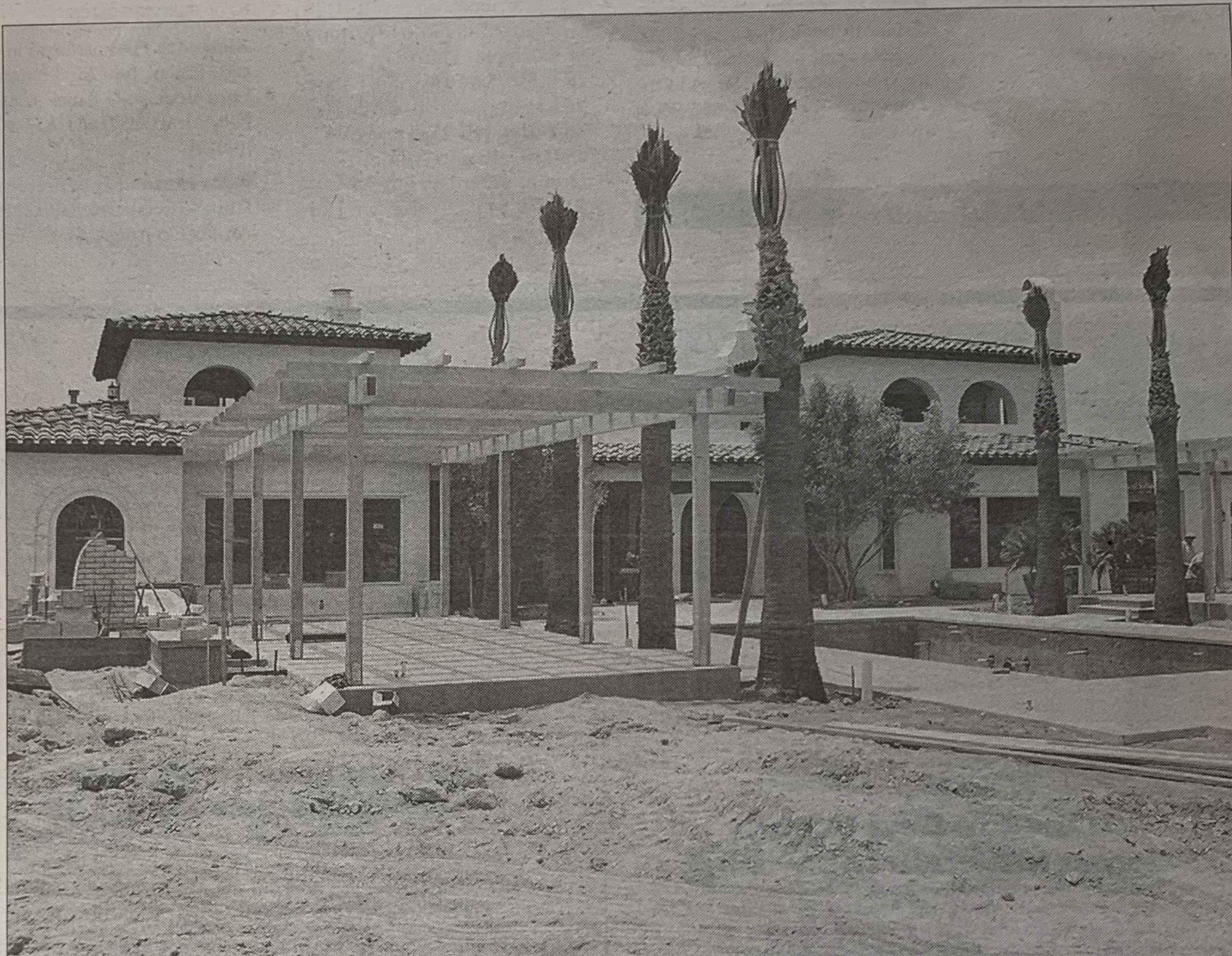
Eastlake home under construction
